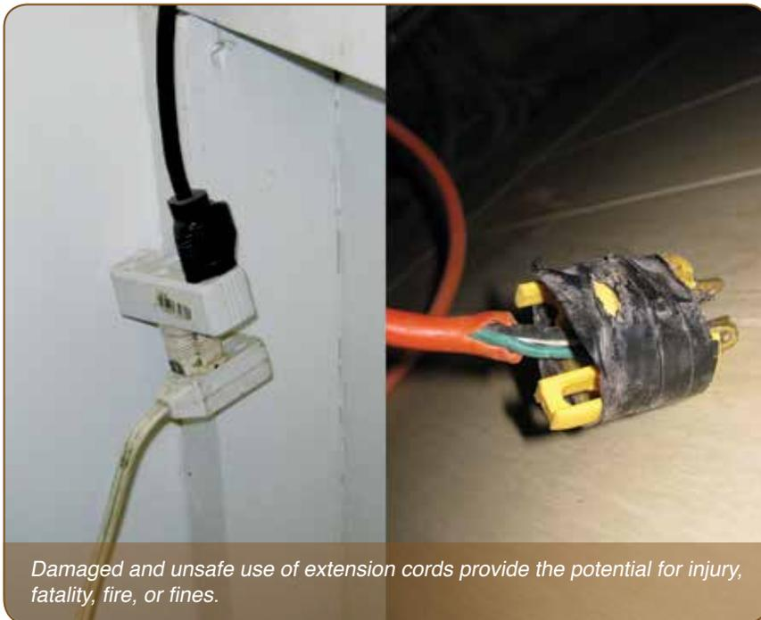
OSHA to find and fine you. Check for corroded prongs and outlets, an issue that is especially prevalent in fertilizer plants and other corrosive environments.
